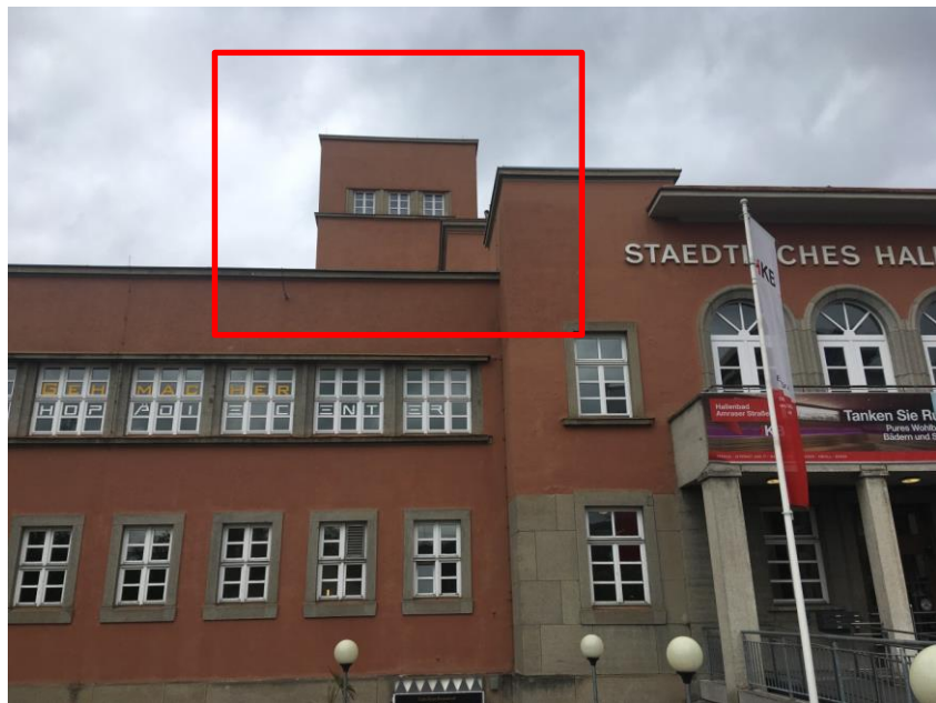
Figure 4: Tower with heat storage in the public swimming pool
