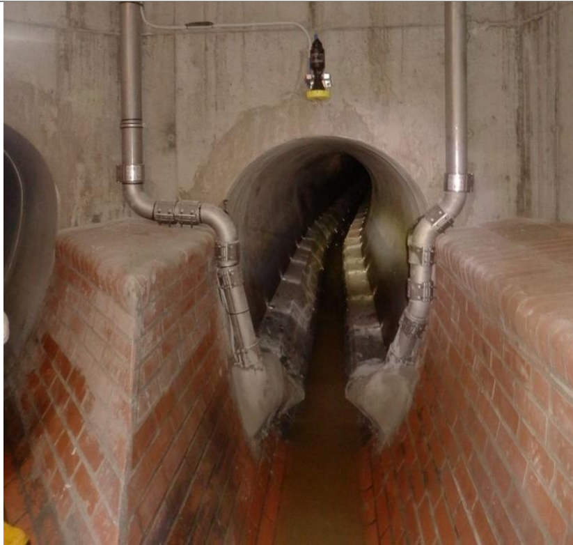
figure 5: Inline heat exchanger for sewage water
