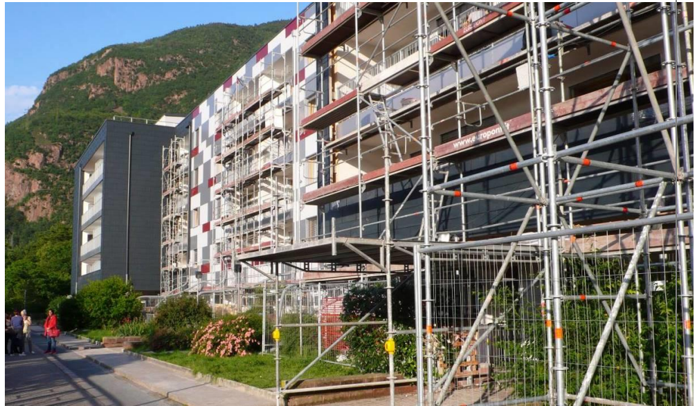
Mounting of the aluminium cladding (photos by Arch. Alberto Olivotto/Arch. Manuel Benedikter)
