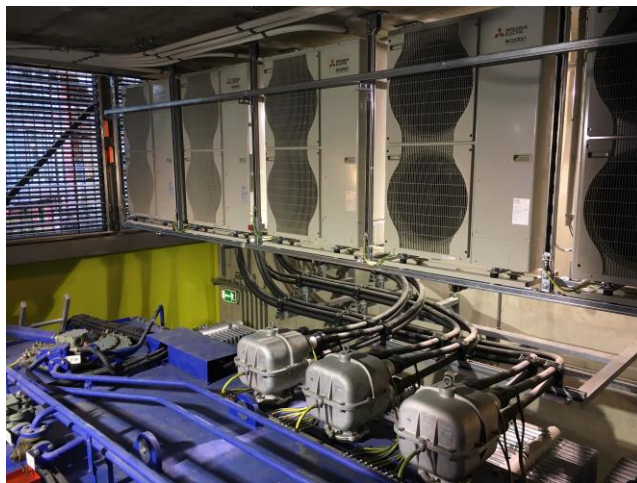
Figure 2: outdoor units of the air-water heat pumps
