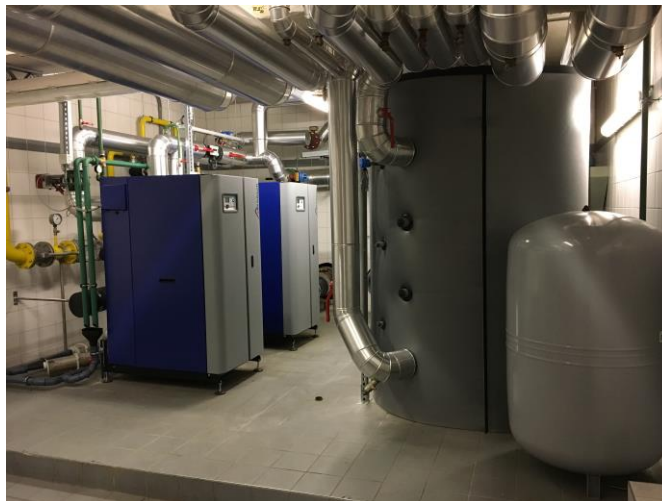
Figure 4: natural gas hot water boiler for peak load coverage
