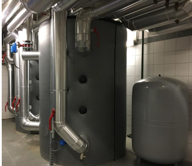
Figure 3: two heat storage tanks with 4,000 litres capacity
