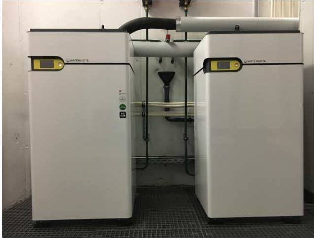
Figure 1: indoor unit of the air-water heat pumps
