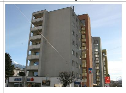
IN40 stock is a typical building block constructed in the second half of the 20th century with related challenges regarding insulation, electric cables, low performing windows, uninsulated roofs and cellars.
