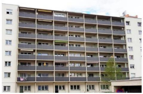
Thermal renovation of the walls, the ceiling, the roof and the windows with triple-glazing. Balconies were completely replaced by new thermal bridge-free ones. Decentralised, flat-specific ventilation with heat recovery was integrated.
