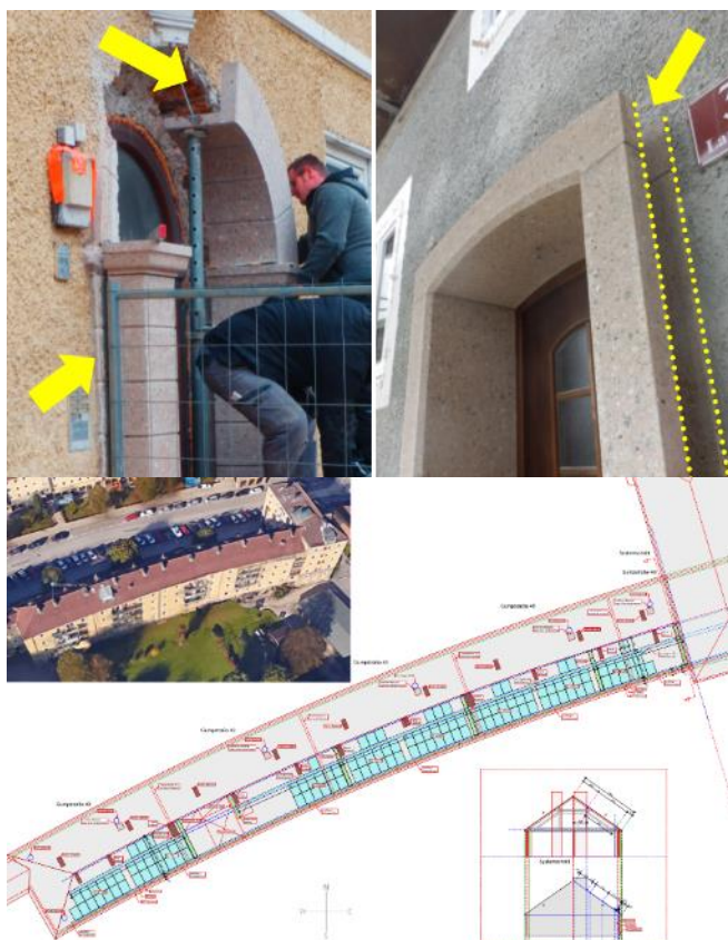
FIGURE 32: IN 3 – RECONSTRUCTED STONE PORTAL WITH SPACE FOR INTERNAL INSULATION (YELLOW ARROWS)
