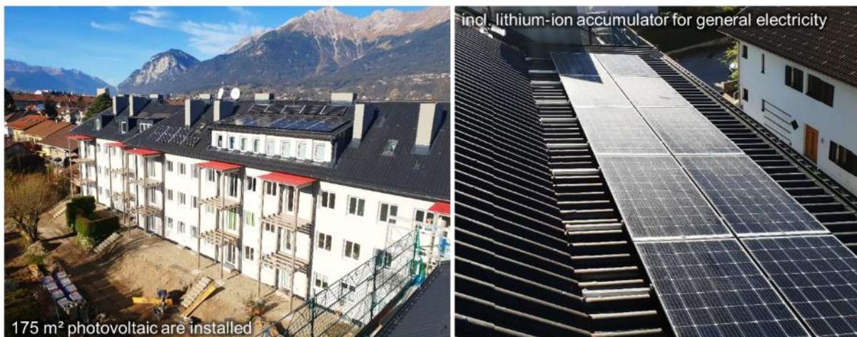
FIGURE 22: IN 22 &amp; 23 – PV-SYSTEM
