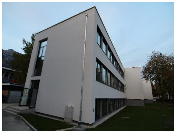
FIGURE 8: VS NEUARZL – AFTER REFURBISHMENT
