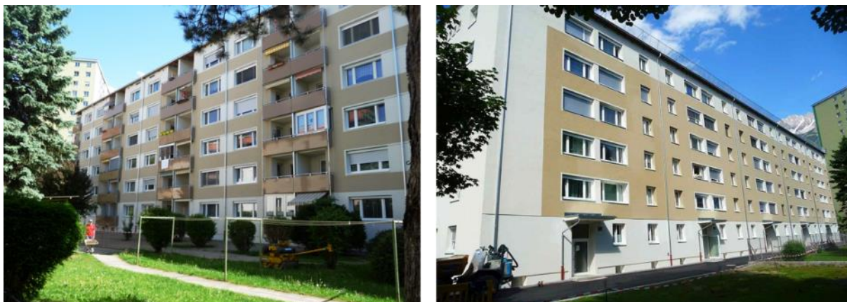
FIGURE 30: IN 43 – AFTER REFURBISHMENT
