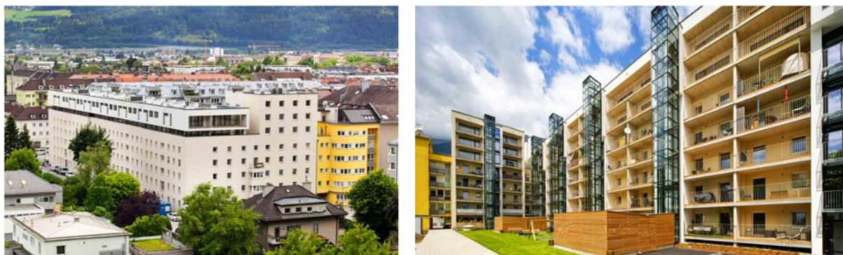
FIGURE 16: IN 13 – AFTER REFURBISHMENT
