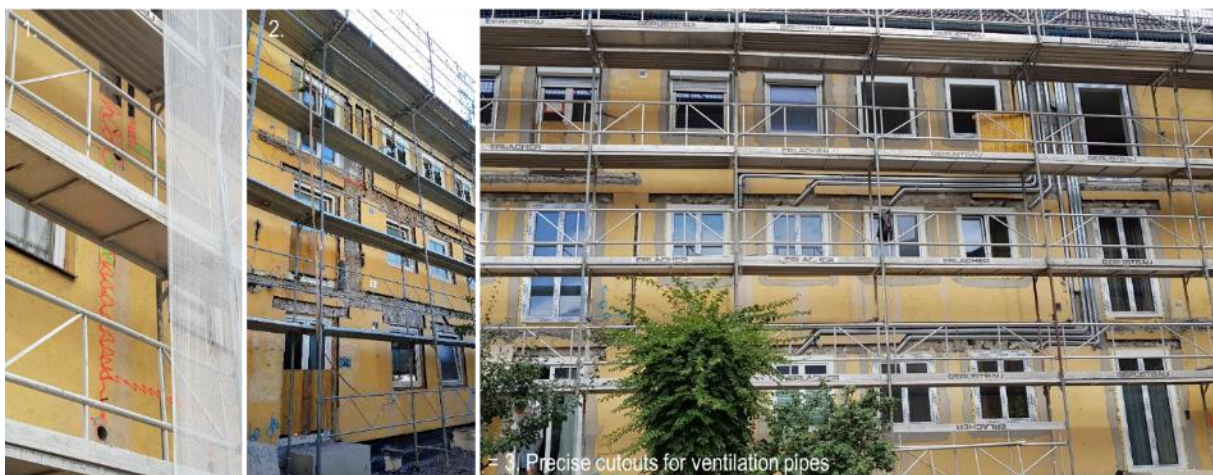
FIGURE 57: BEST 12 – 3 STEPS OF INTEGRATION OF ROOM WISE AIR DISTRIBUTION INTO THE THERMAL SHELL
