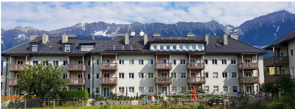
FIGURE 26: IN 22 & 23 – AFTER REFRUBISHMENT
