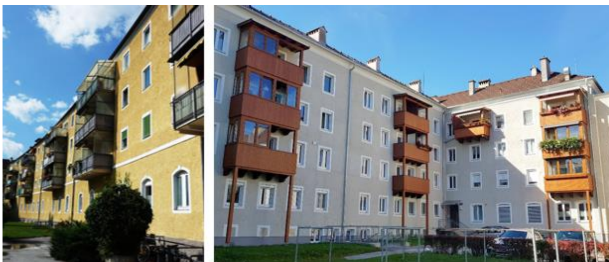
FIGURE 35: IN 3 – REFURBISHMENT OF LOCAL CULTURAL HERITAGE; BEFORE & AFTER
