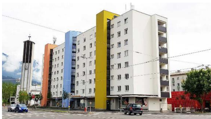
FIGURE 13: IN 40 – AFTER REFURBISHMENT
