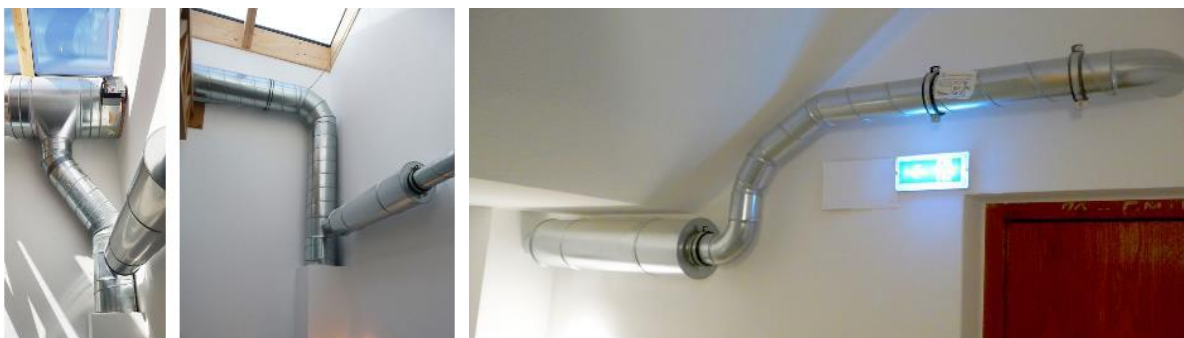
FIGURE 29: IN 43 – CENTRAL AIR DISTRIBUTION OF VENTILATION SYSTEM WITHIN STAIRCASES
